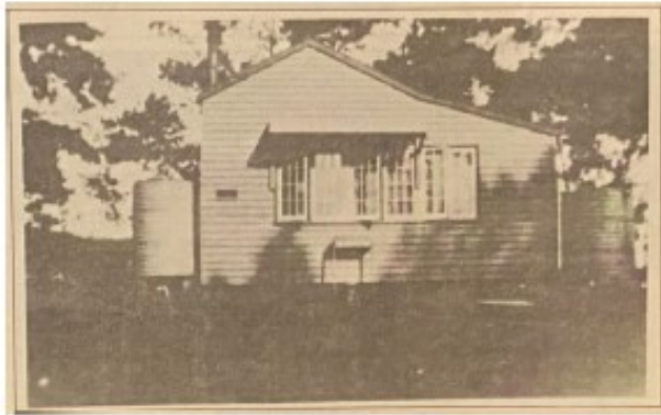
The school just before it was moved.
